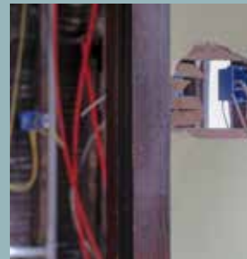
February 2019 – Electrical work complete.
