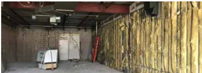
Early March 2019 – Demo complete. Ready for walls, flooring and a ceiling!
